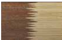
IRREGULAR finger joint Aboutage enture irrégulière
